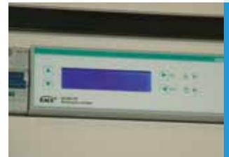
An ekinex® KNX mixing actuator controls the servo motor of a mixing valve delivering the correct temperature to the fan coil circuits
