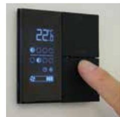
End users can modify the setpoint of  $\pm 2^\circ\text{C}$  and manually control the fan speed
